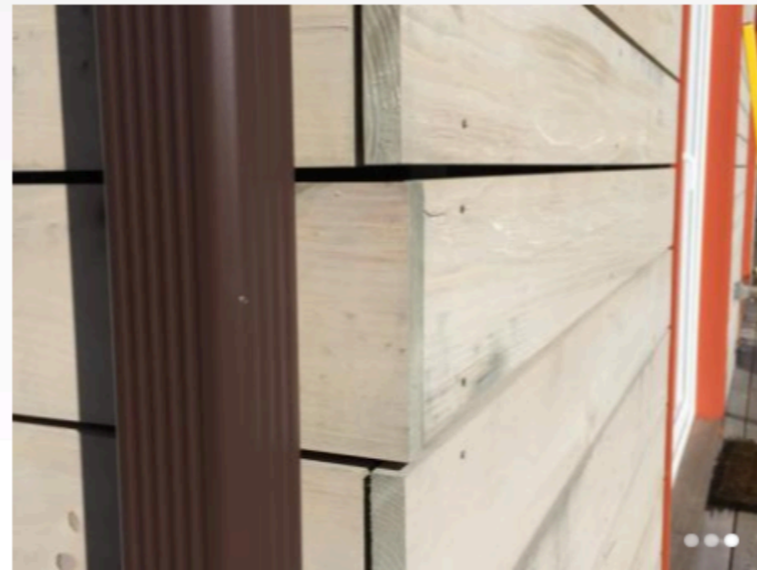
Mechanic Street Passive House rainscreen detail
