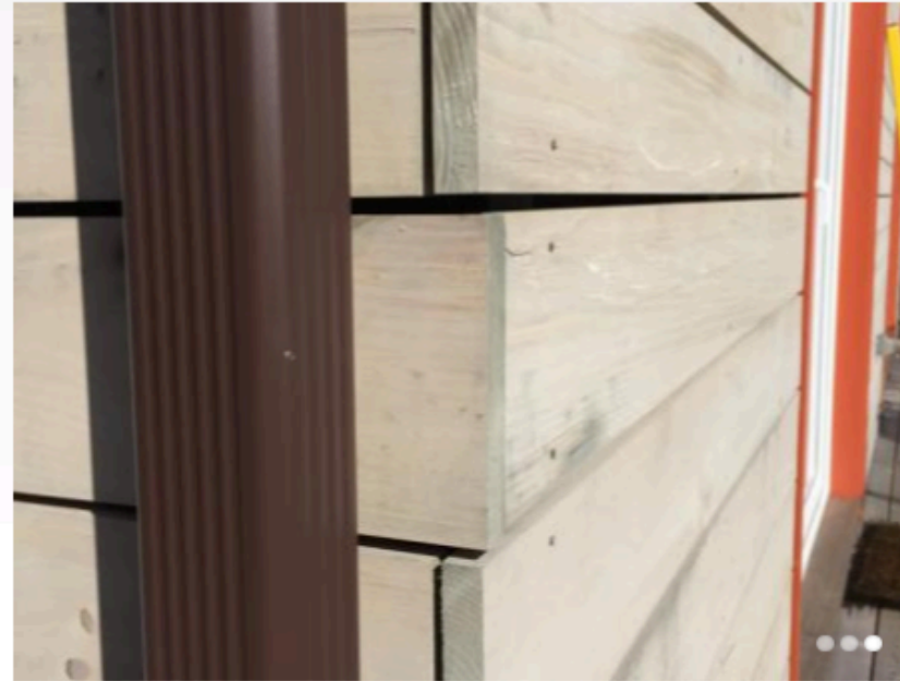
Mechanic Street Passive House rainscreen detail
