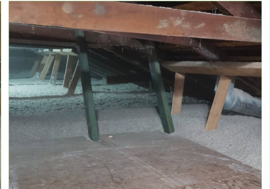
Insulated attic with a framed-up plywood mechanical platform
