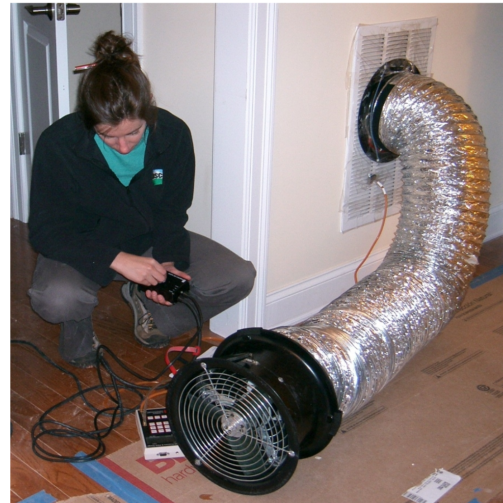
Duct Leakage Test
